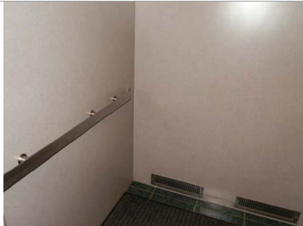
Interior elevator wall finishes
