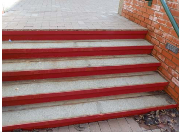
Concrete steps evidencing deterioration
