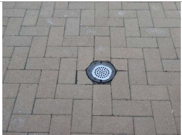
Drain in courtyard
