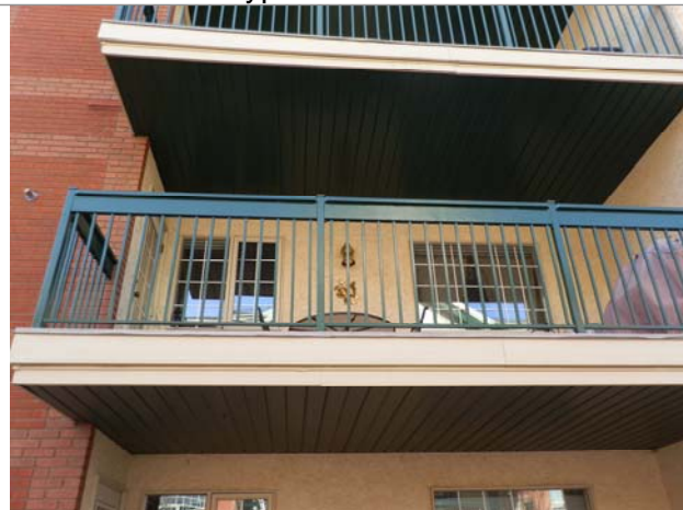
Balcony fascia and railings
