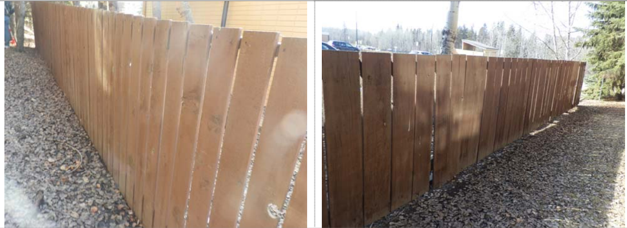
Wood fencing on west side of property
