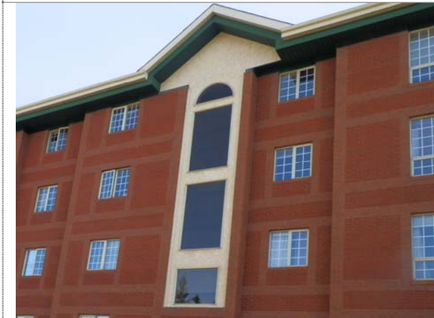
Stairwell & unit windows
