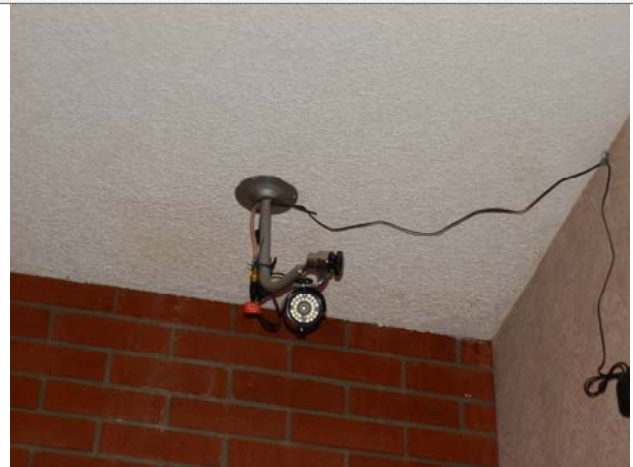
Camera attached to intercom system
