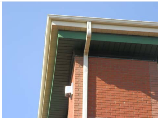
Typical eavestrough/downspout connection
