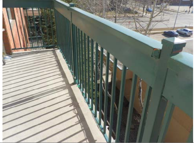
Balcony railings with metal capping
