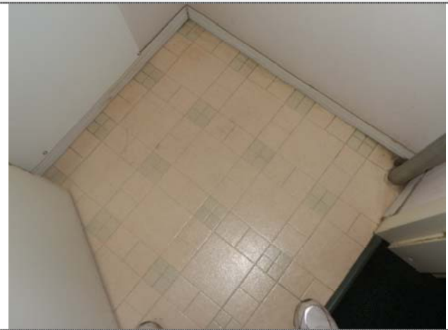
Linoleum in garbage chute room
