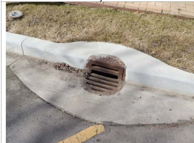
Drain in roadway
