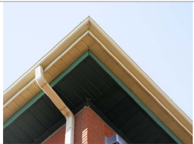
Soffit at roof overhang
