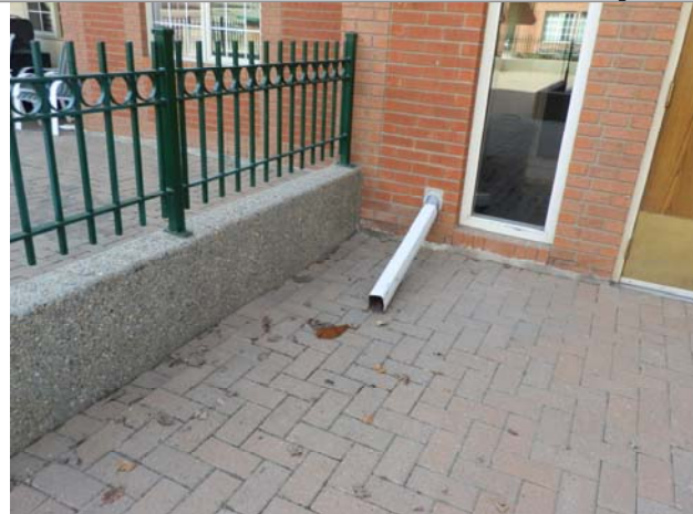
Brick unistone, concrete curb & wrought iron fence
