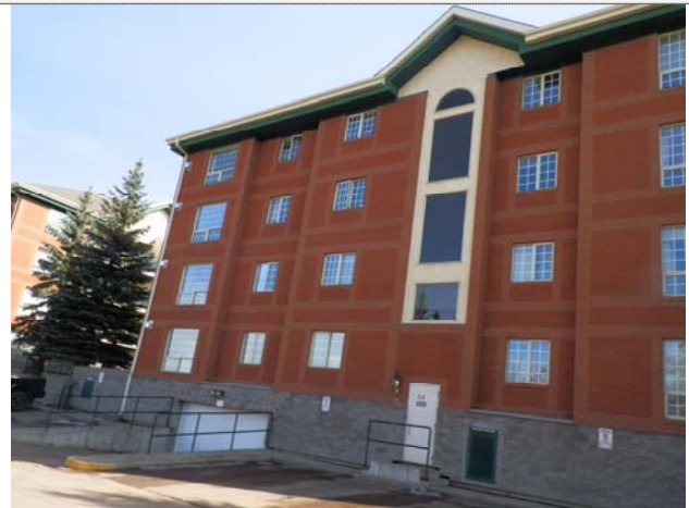
Side of building
