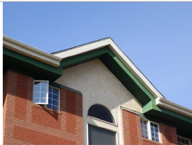
Fascia at roof termination
