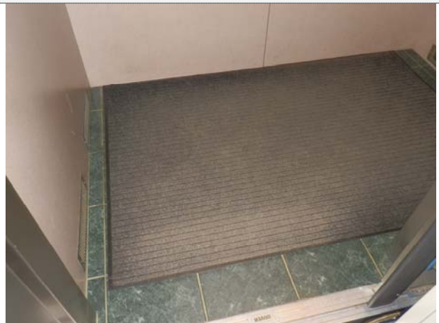
Interior elevator flooring finishes
