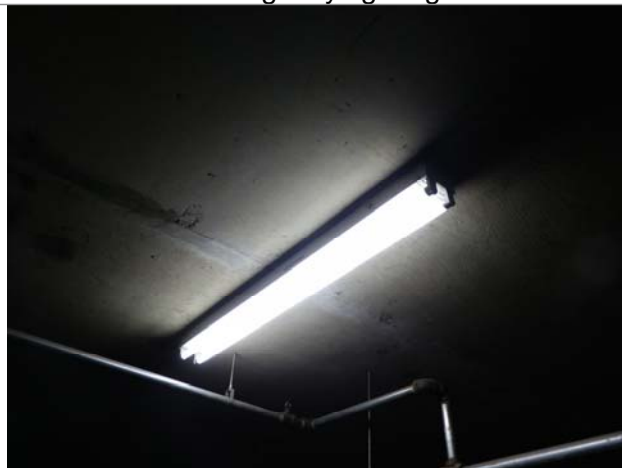
Parkade florescent lighting
