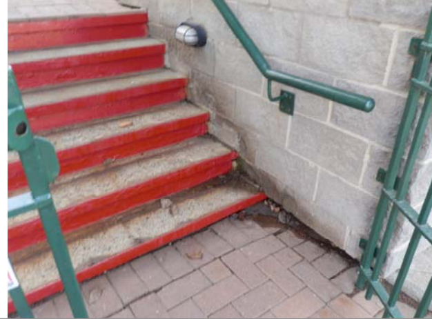
Concrete steps evidencing deterioration
