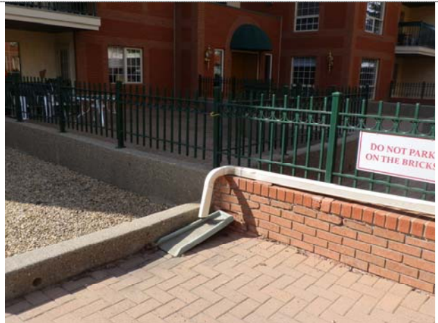
Brick and concrete walls/curbs with wrought iron fencing
