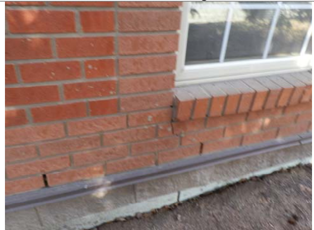
Damaged brick
