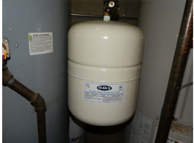
Small expansion tank Pro Flex 2 - M: PH25
