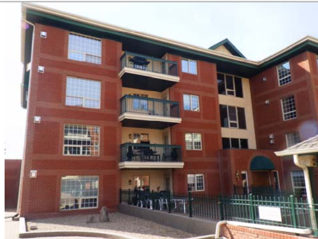
Front of building
