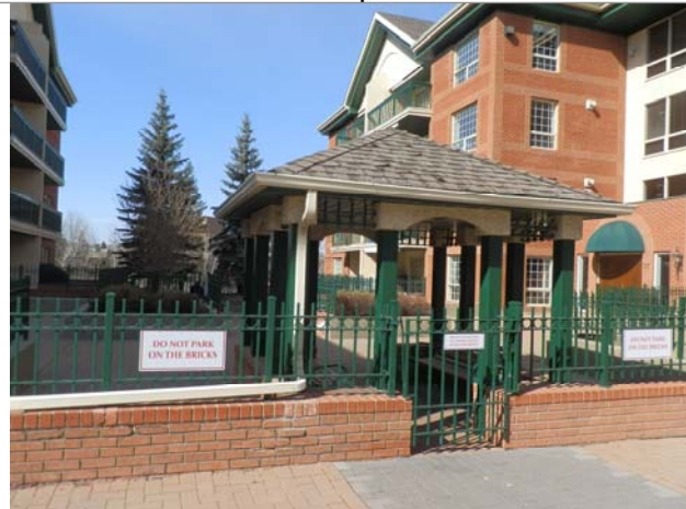
Gazebo entrance and wrought iron fencing
